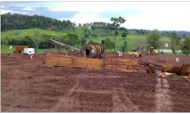
Photo 1: A: Trommel, B: Permitted water source, C: Generator, D: Water Pipeline, E: Temporary Tailings Dam and F: Hopper. (CNW Group/Meridian Mining S.E.)
